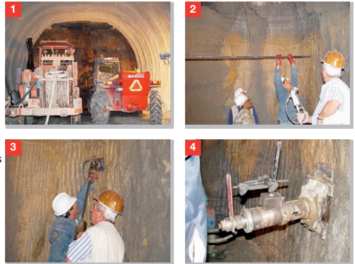
1 Excavation works; 2 – 3 Installation of Omega-Bolt® 4 Bolt Testing
